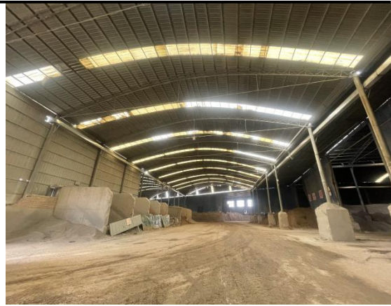
喷淋洒水抑尘
